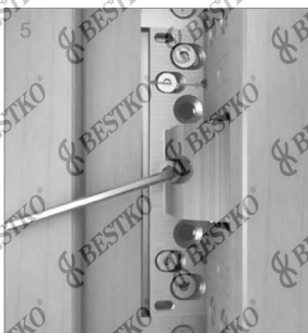
5. Correct the alignment by adjusting by adjusting socket screw on hinge body.
