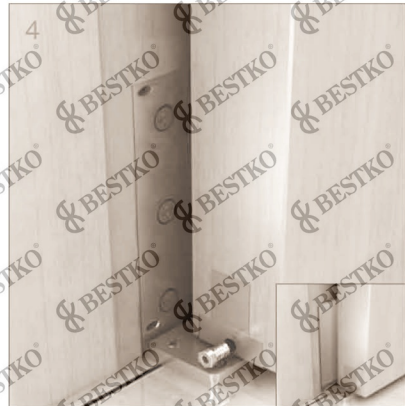
4. Remove the set screw (for hold open version only), fix the cover plates properly and installation is done.
