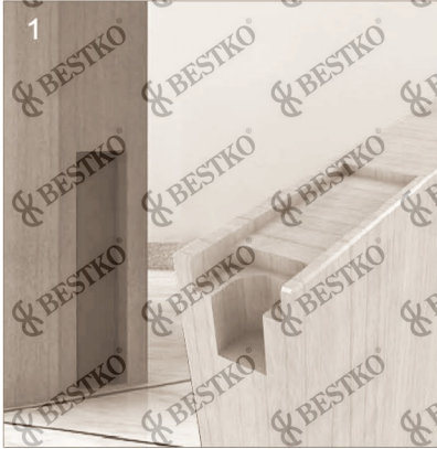
1. Prepare notches on door leaf and door jamb with template provided.
