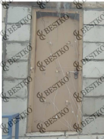
Fig. 6 – Unexposed Side after 90 Minutes
